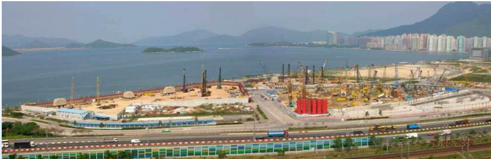
Progress in July 2009
