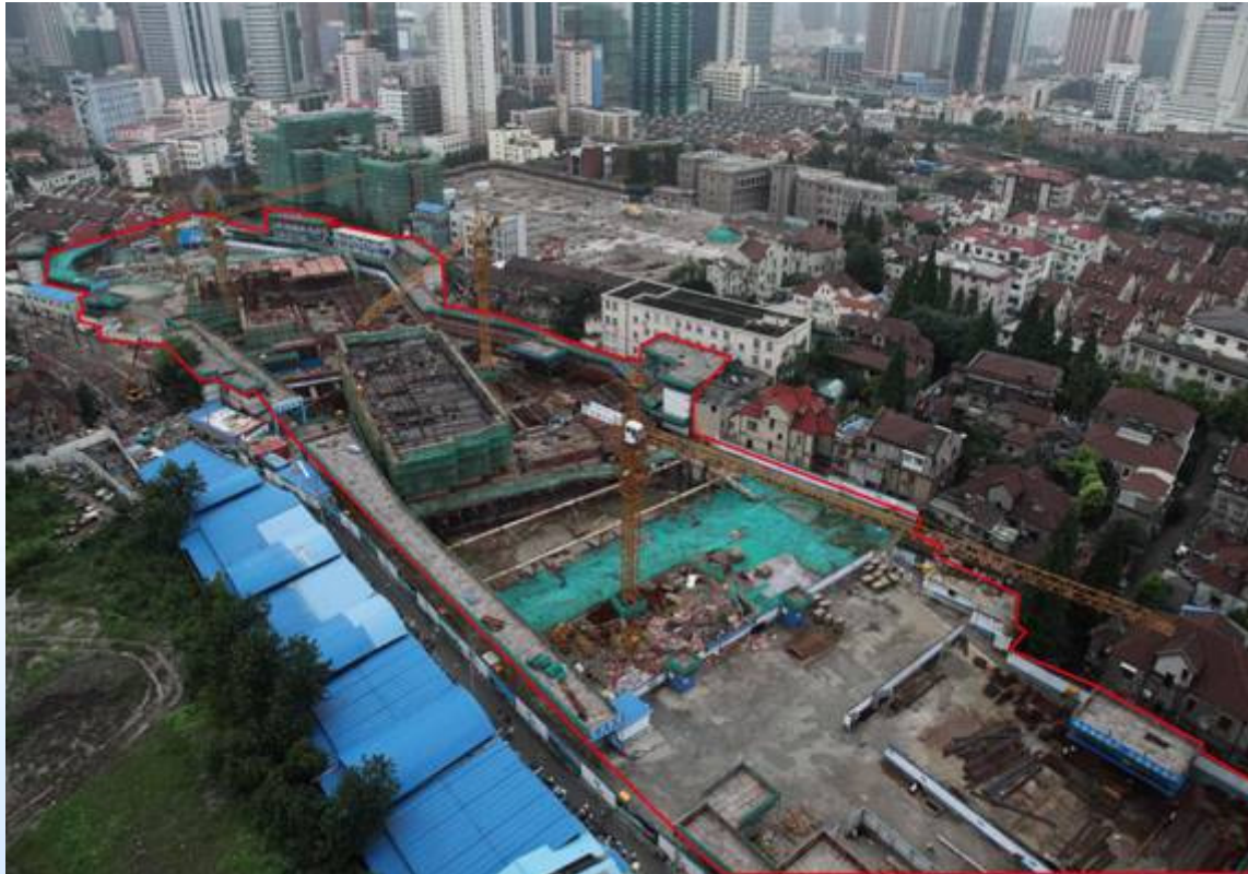
Progress in August 2009
