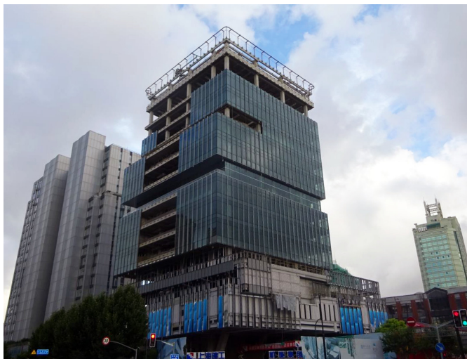
Shanghai Office project, Jingan District
